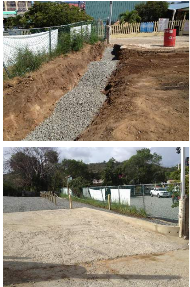
Figure 46. Gravel filter and parking lot stabilization by PDC in Parguera, Puerto Rico.
