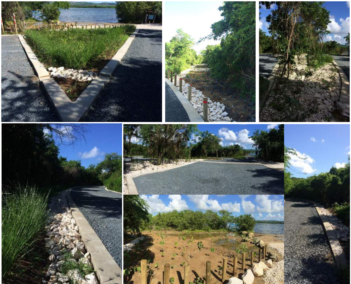
Figure 37. BMPs implemented following a train treatment approach in Mosquito Bay in Vieques Puerto Rico. Practices include bioswale, bioretention, raingardens, constructed treatment wetlands and permeable parking.
