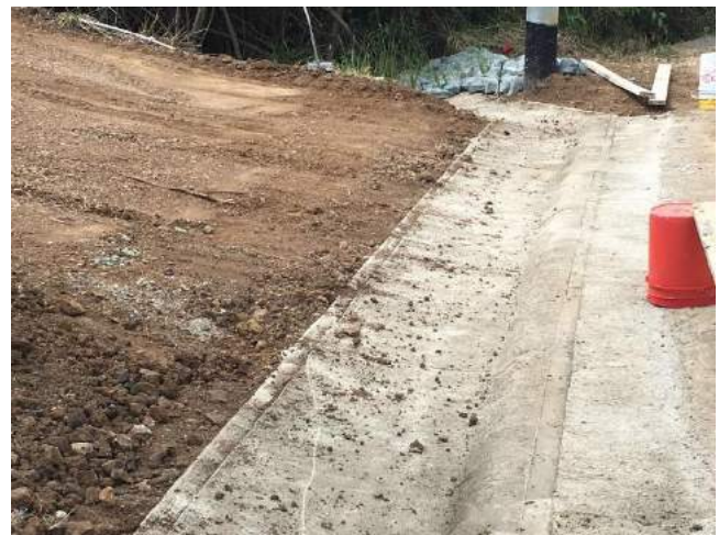
Figure 59. Example of swales made by PDC in Culebra (concrete) and in a coffee farm (stones).
