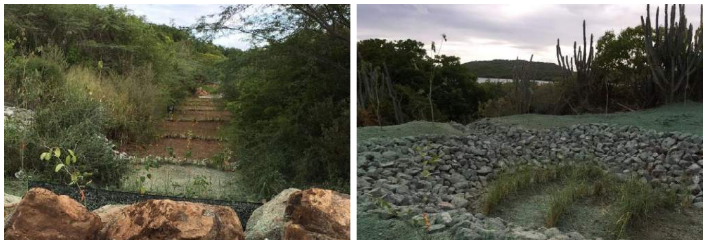
Figure 41. BMPs implemented following a train treatment approach in Puerto del Manglar in Culebra, Puerto Rico. Practices include bioswales and sediment traps.
