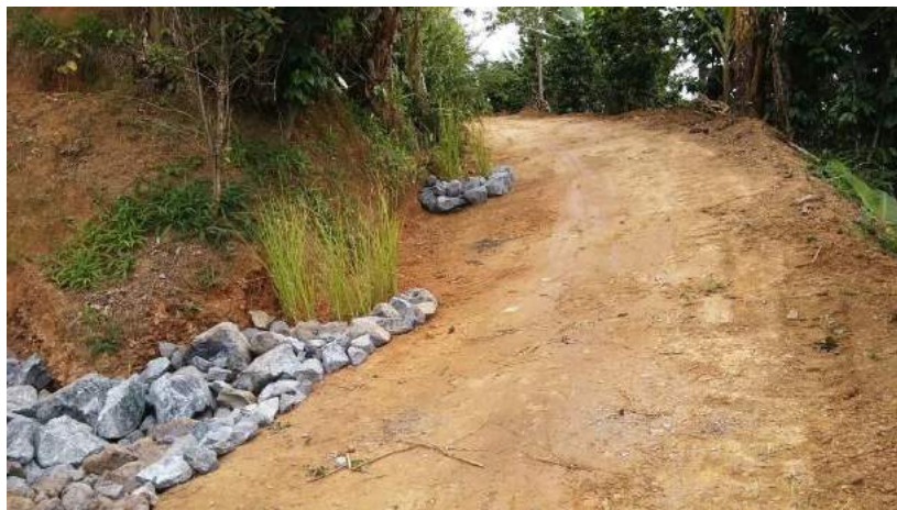
Figure 54. Example of check dams constructed by PDC on a dirt road network in coffee farms of Yauco Puerto Rico.
