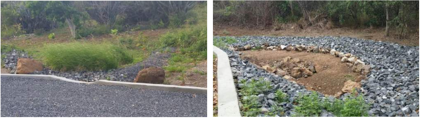
Figure 39. BMPs implemented following a train treatment approach in Punta Soldado in Culebra, Puerto Rico. Practices include bioswales, bioretentions, raingardens, sediment traps and permeable parking.
