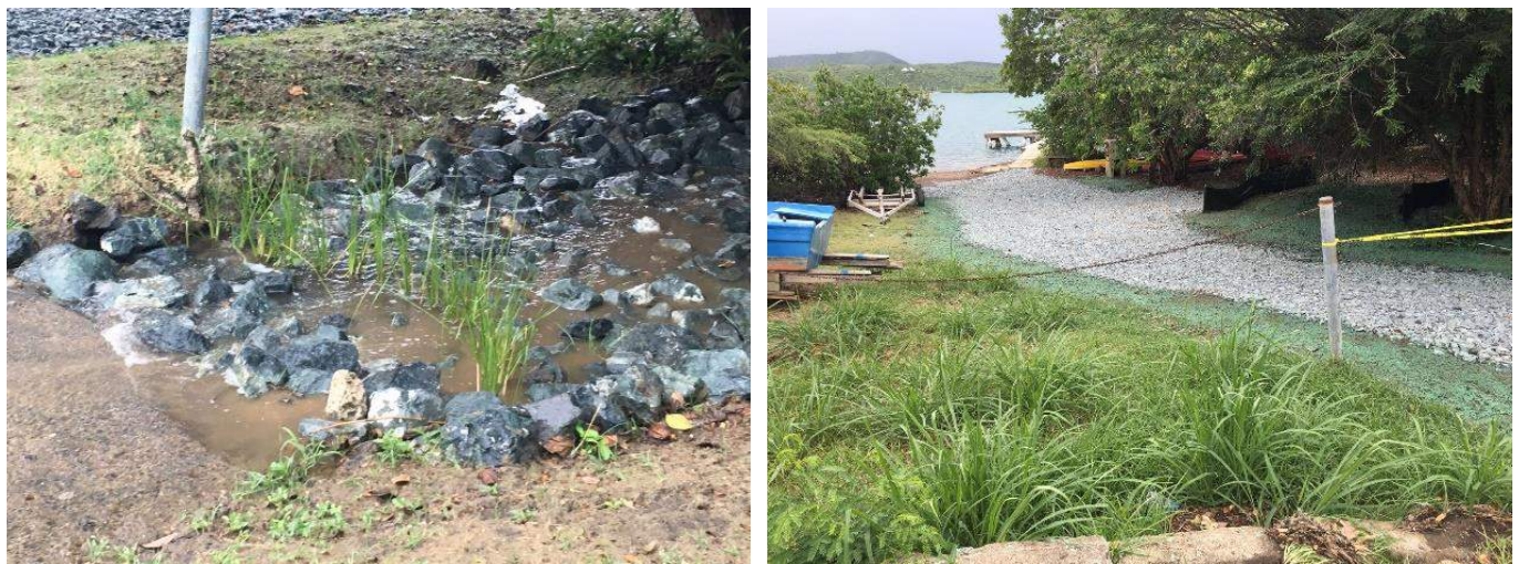
Figure 40. BMPs implemented following a train treatment approach in Fulladosa Culebra, Puerto Rico. Practices include bioswales and raingardens.
