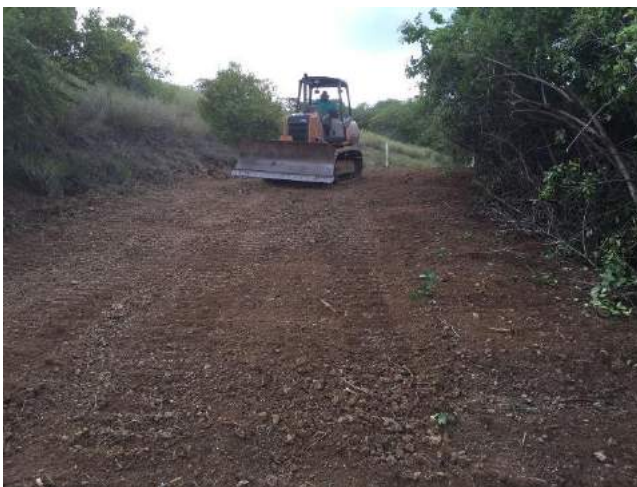
Figure 53. Example of regrading and compaction by PDC on a dirt road in Culebra, Puerto Rico.
