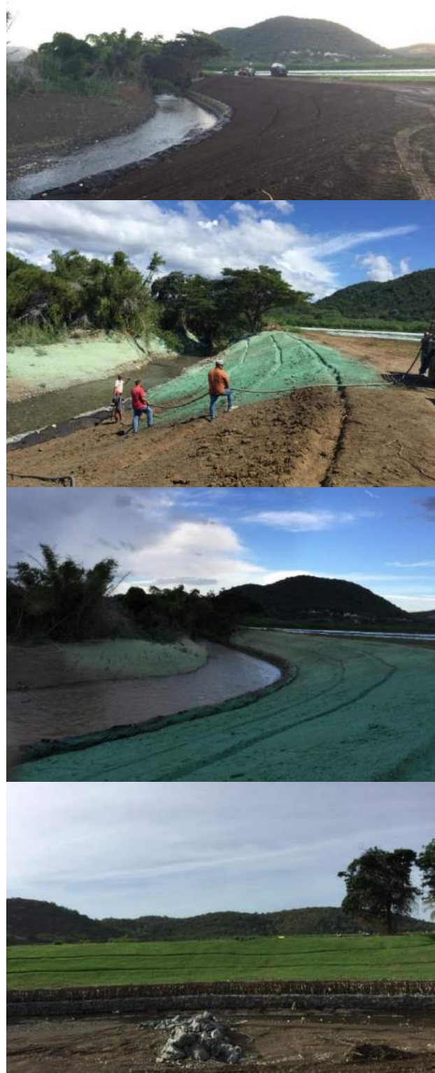
Figure 52. Hydroseeding implementation by PDC on a riverbank stabilization project in the Río Loco, Guánica Puerto Rico
