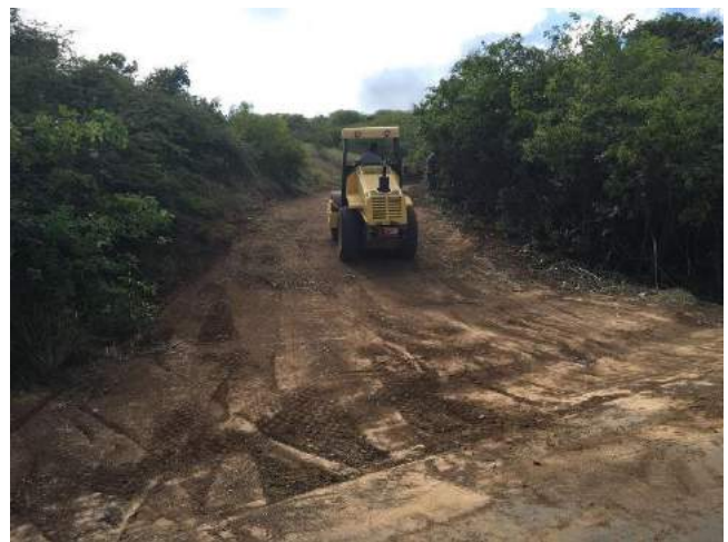
Figure 53. Example of regrading and compaction by PDC on a dirt road in Culebra, Puerto Rico.
