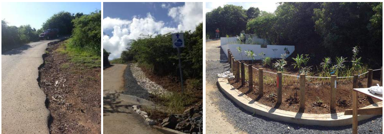
Figure 38. BMPs implemented following a train treatment approach in Zoní Beach at Culebra Puerto Rico. Practices include bioswales, bioretentions, raingardens and permeable parking.
