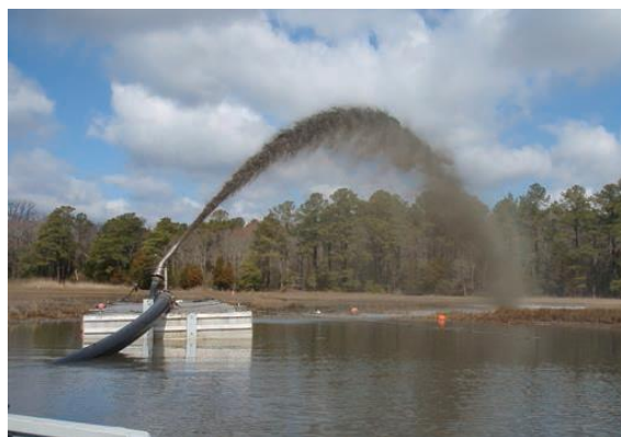
Photo 1. Accommodate Case: Dredged Material Reuse Pilot Project. Sediment dredged from Pepper Creek Near Dagsboro in Sussex County, Delaware, used to elevate marsh surfaces.
