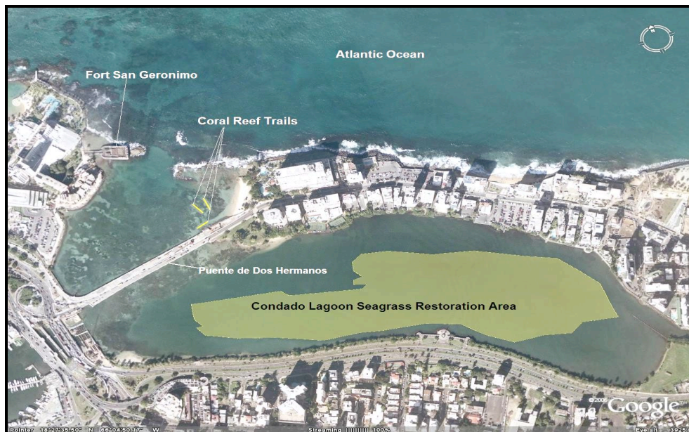
Aerial view of the Seagrass Restoration and Coral Reef Trail Projects in Condado Lagoon, San Juan, Puerto Rico.
