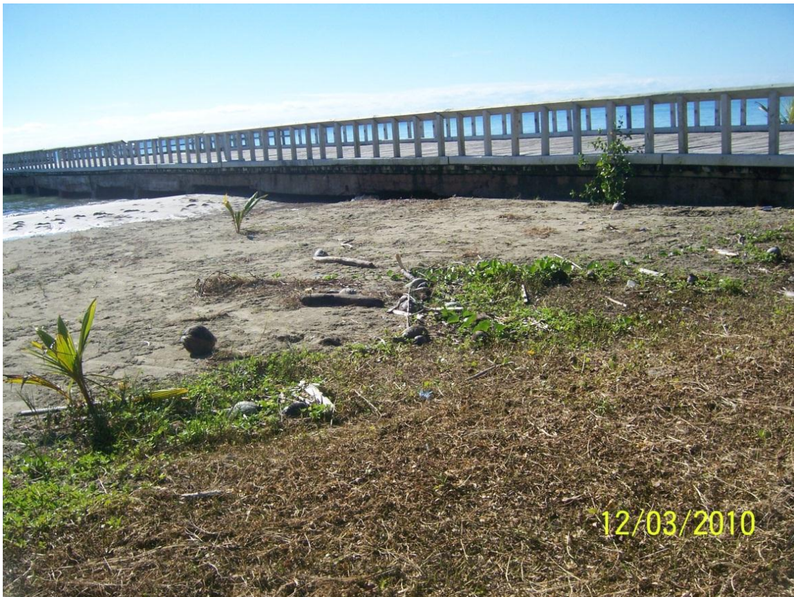
Figure 56. Dock structure located to the southward station 2.
