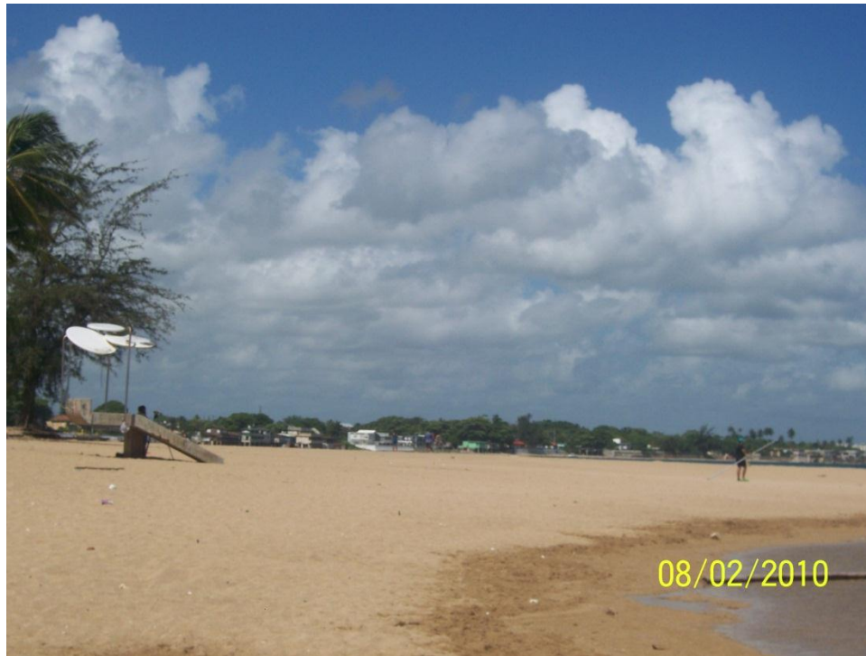
Figure 34. Beach profile 1 at Playa Puerto Nuevo (August 2010). This barrier protects the station from waves approaching from northwest.
