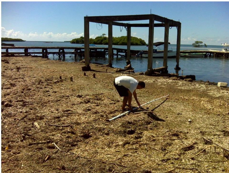
Figure 82. The dock located between station 1 and 2 apparently do not block sediment transport to the west. This dock was build-up with an open base that may do not block sediment transport.
