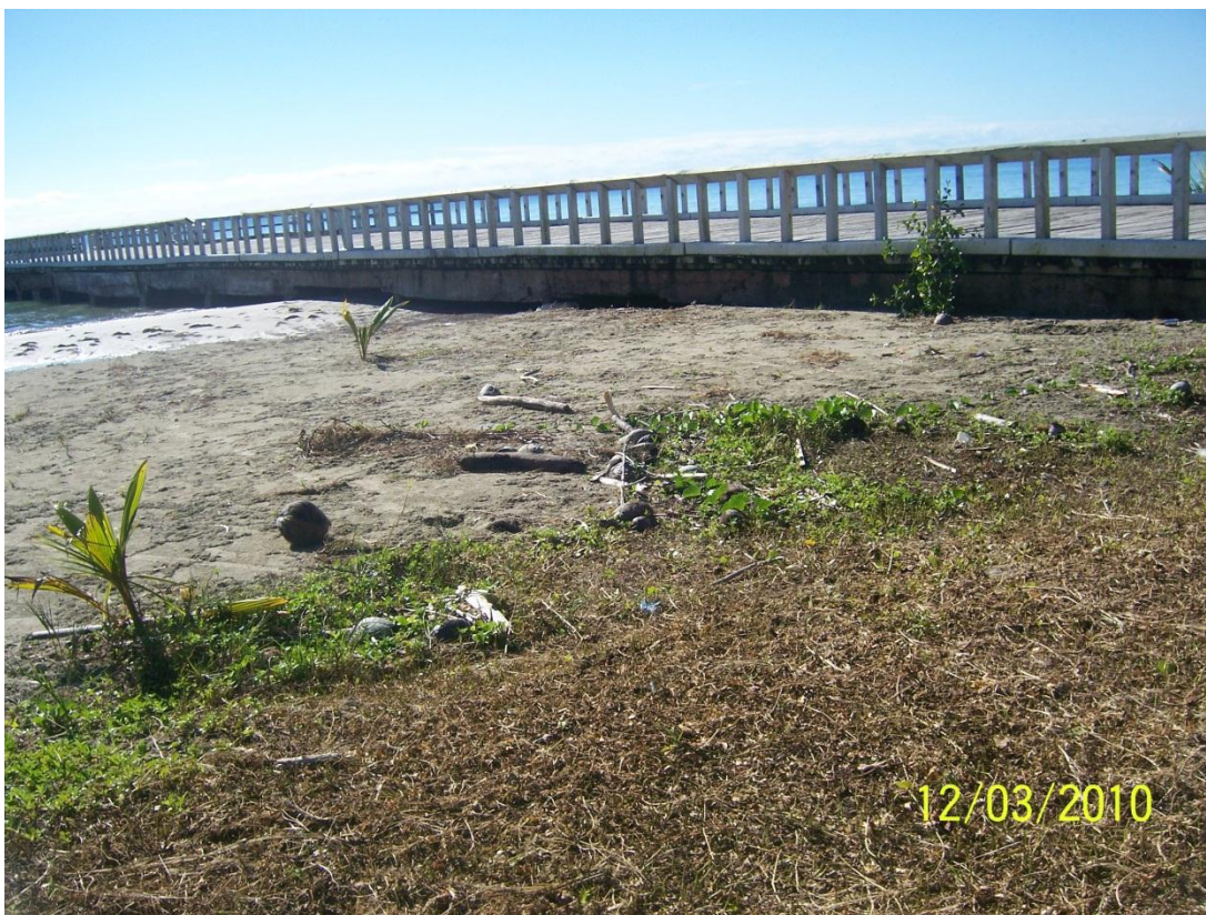
Figure 78. Beach profile Station 2 at Playa Humacao. The dock apparently blocks sediment transport to the south (beach station 1).
