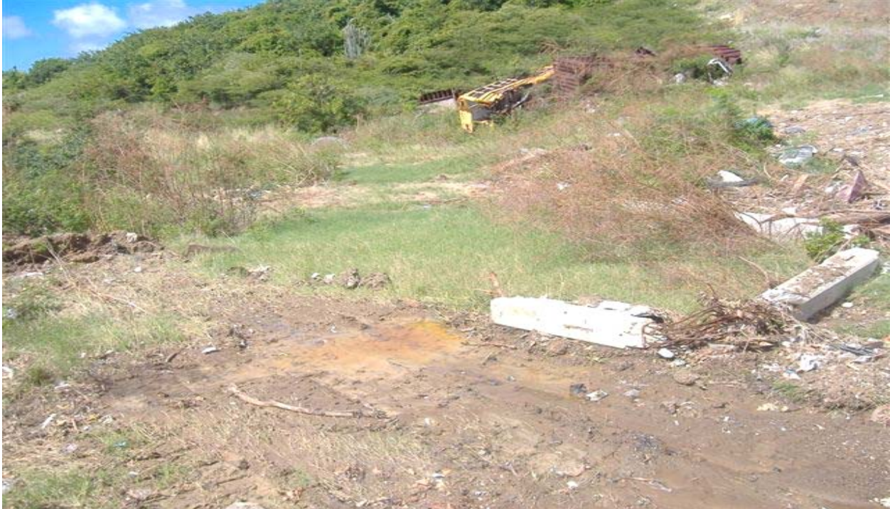
Photographs No. 18 & 19- Looking to the north. Leachate Zone Z-2 which is closed to the area facing the Luis Peña Canal. Any water runoff control was observed along this zone creating the possibility of leachate migration to the Reserve. The leachate leakage was observed very clearly in Photo No. 17 below.
